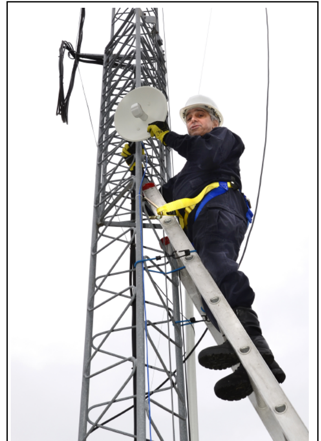
K3RF aims microwave dish on ARES tower at repeater link dish on Fair Acres.
